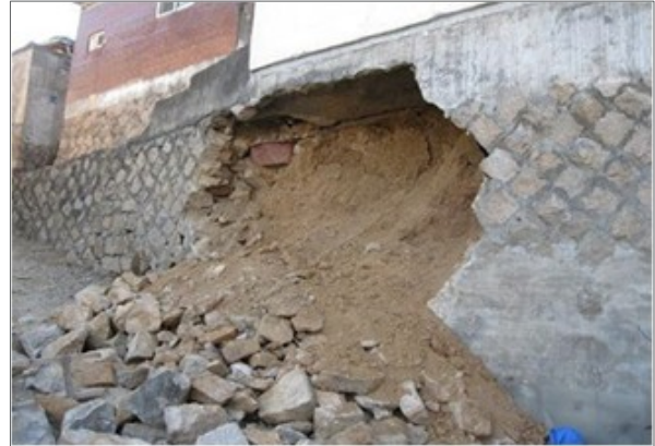
Figure 11 - Collapsed Stonework
