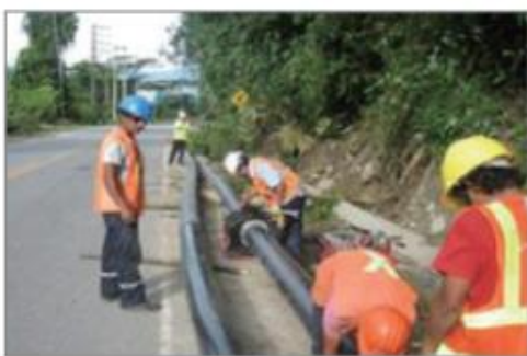
Upgrading the water pipe network
