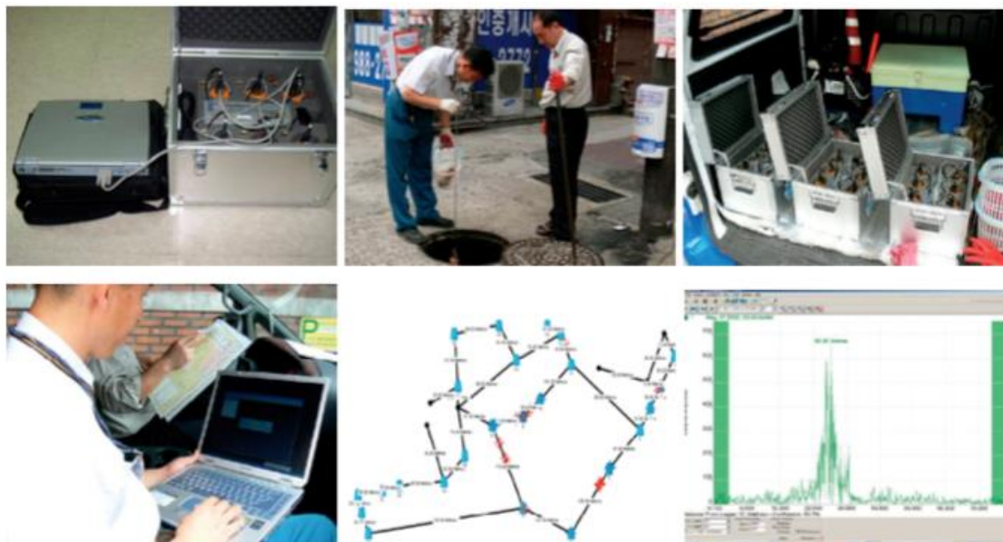
Figure 8. Leak detection using multipoint leak noise correlator
