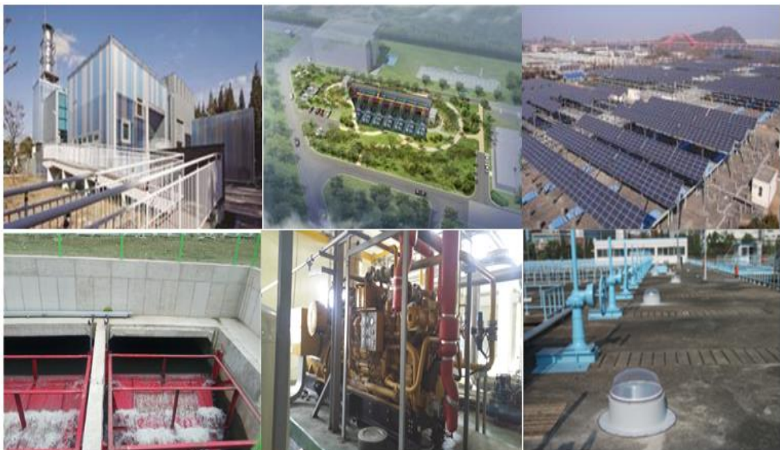
Figure 11. New and renewable energy producing facilities in WWTPs in Seoul [Clockwise from the top left, combined heat and power plant (Seo Nam), recovered heat supplying unit (Tan Chun), Photovoltaic power plant (Seo Nam), small hydropower plant (Seo Nam), Power plant using biogas (Seo Nam), natural lighting for underground utility tunnel (Joong Rang)]
