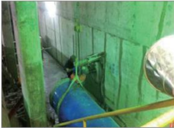
Perforating works for pipes connected to the ground
