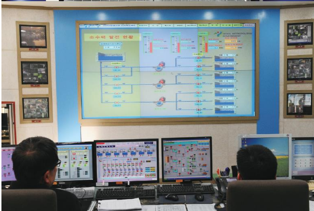
Arisu Small Hydropower plant takes advantage of the kinetic energy of non-pressurized water produced in the Amsa purification center and Noryangjin reservoir. For the first time in Korea, Arisu SHP uses waterwheel installed in the drinking water supply network to produce hydropower.
