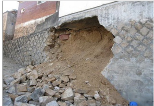
Figure 11 - Collapsed Stonework
