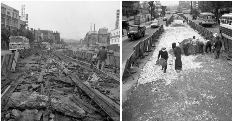
[Figure 12] Demolition of Tram Tracks
